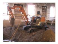
These first two pictures are showing the auditorium area. The floor has been dug up for underground plumbing. The stage has also been removed as it had been a haven for coon.
